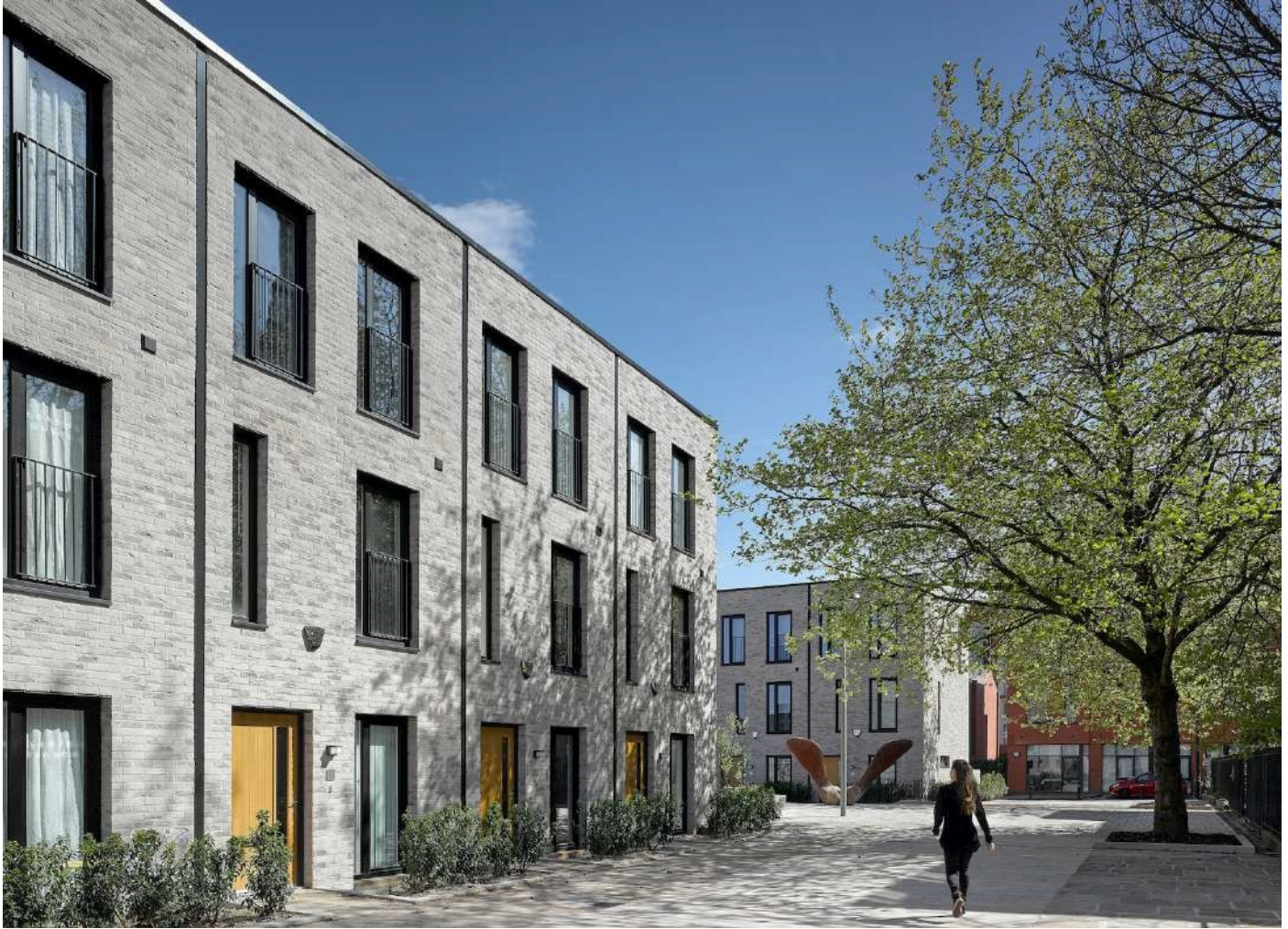
Figure 11 – Street elevation, Timekeepers Square – source: Buttress Architects & Photographer Daniel Hopkinson
