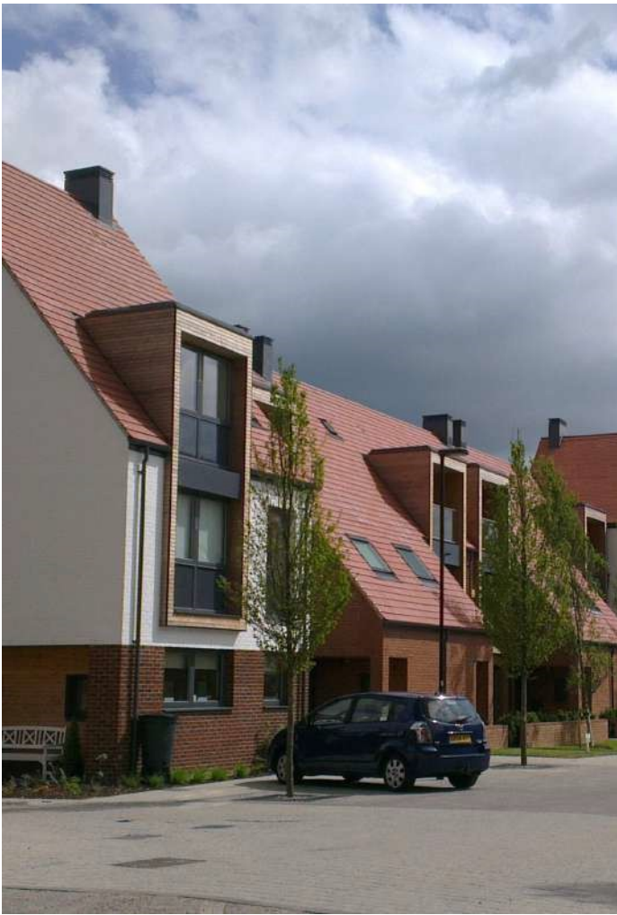
Figure 27 View of Derwenthorpe scheme image credit - Studio Partington
