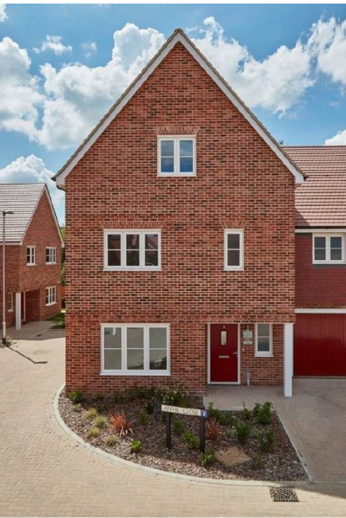
Figure 28 View of Balsham Buildings, Hill Residential Ltd
